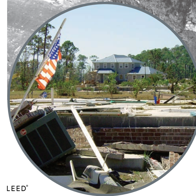
Devastation from Hurricane Katrina - 2005
