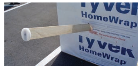
Wood frame wall - severe damage
