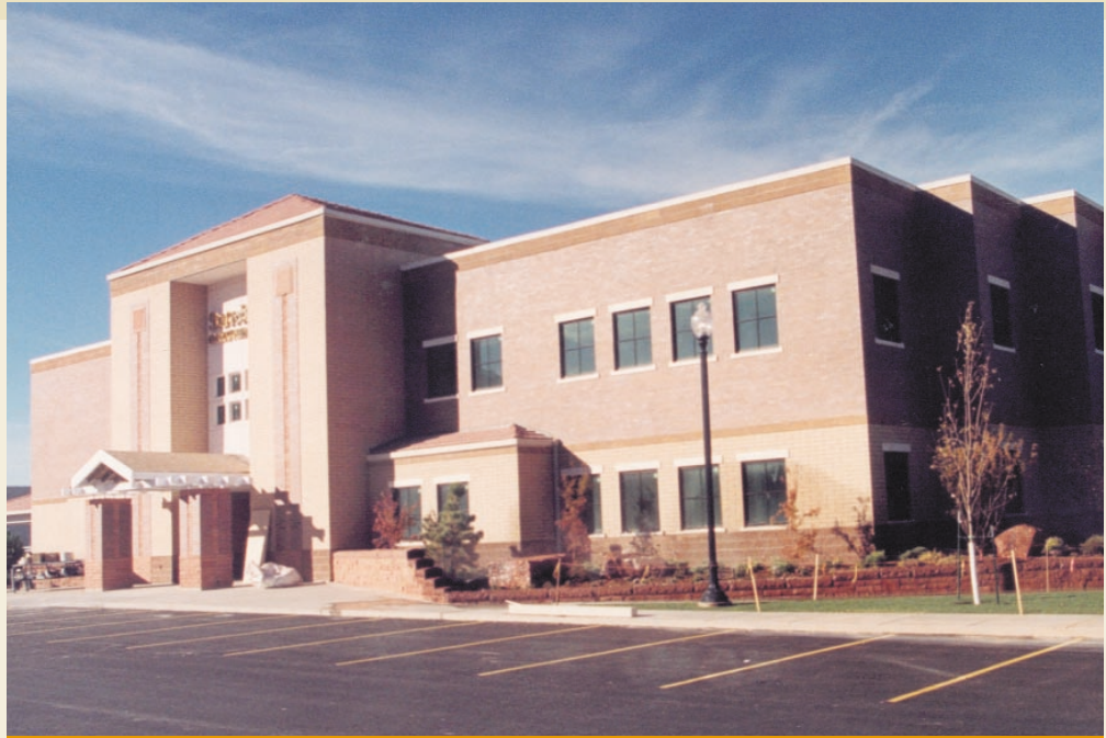
State Bank of Southern Utah, Cedar City, Utah DISTRIBUTOR › Blackburn & Associates
